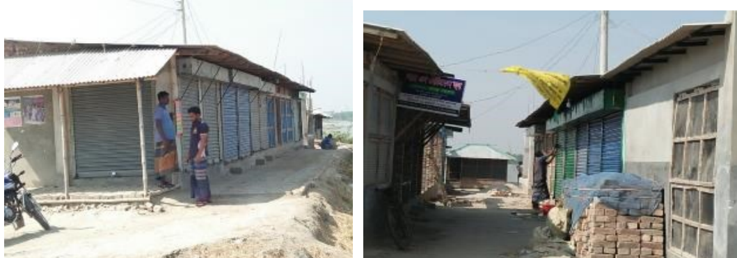
Photo 13: Market Relocation for Joynagar Bazar at Polder 32
